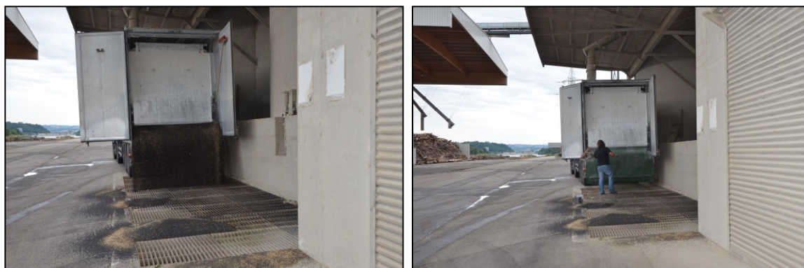
Figure 47: Cleaning of trucks.
